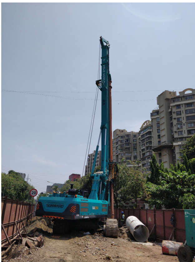
Hydraulic Piling Rigs at Mumbai Metro Line 4
