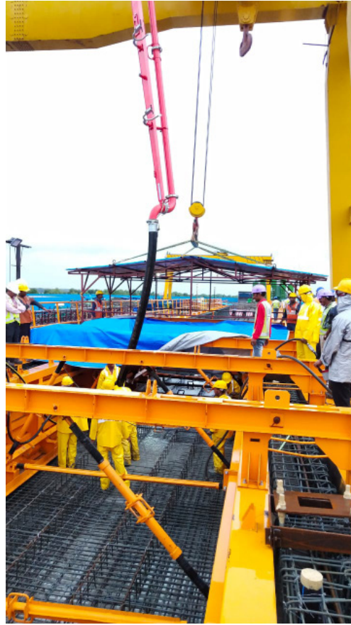
Precast Girder Casting for Mumbai Metro Line 4, Thane
