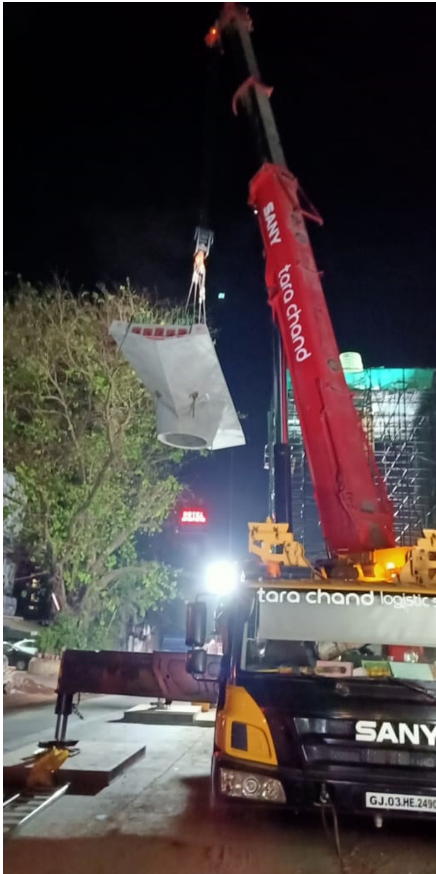
Critical Erection work being carried out for Mumbai Metro Line 4
