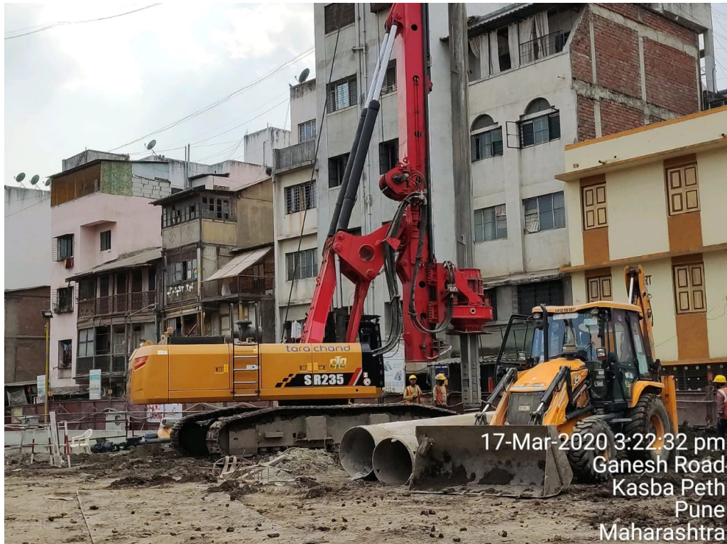
Piling Work in full swing at Pune Metro
