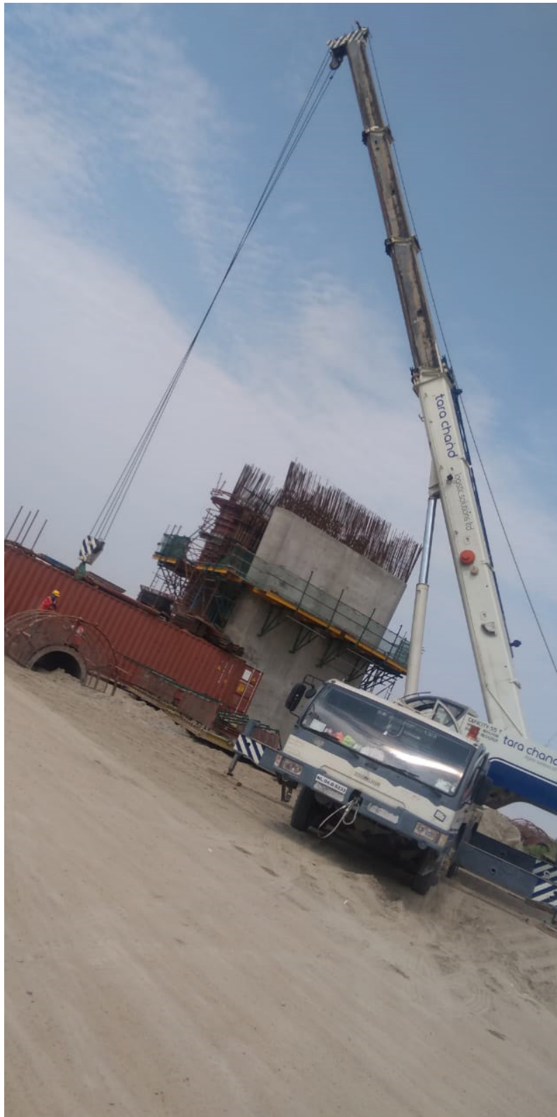
Our 55MT Capacity Crane working by the Ganges River in Bihar
