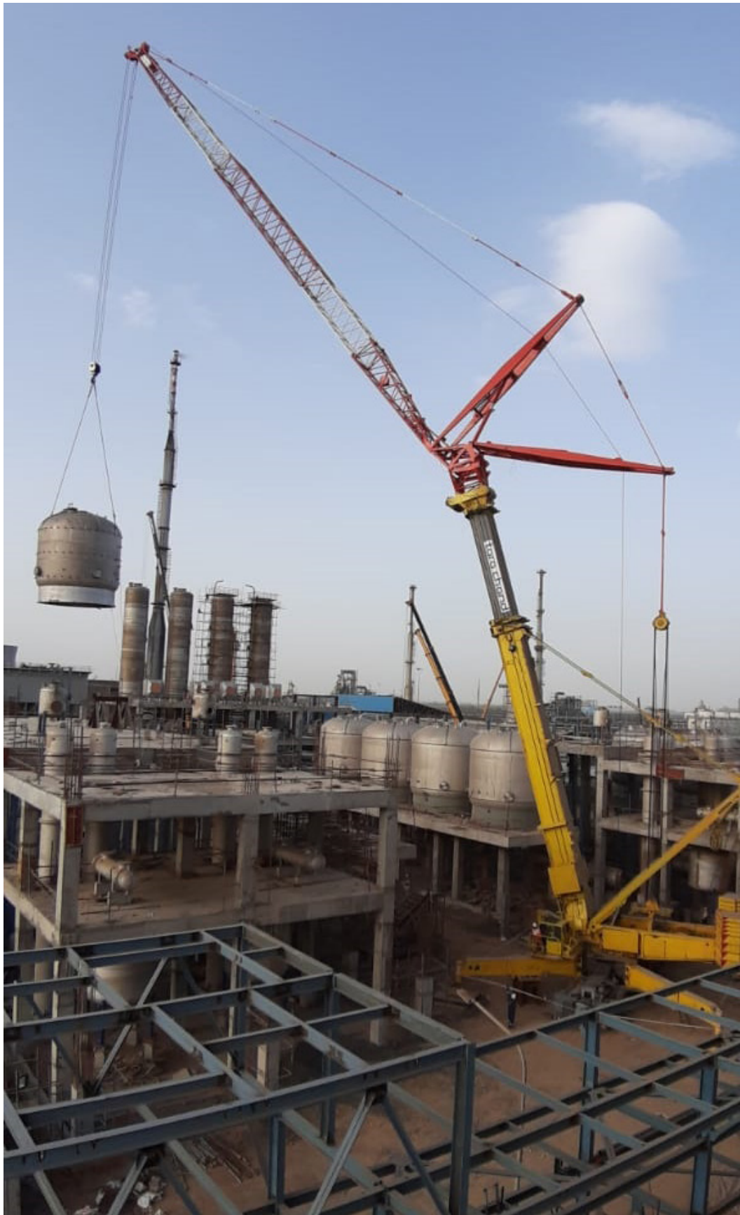
Another critical lift being executed by our 800MT Liebherr LTM1800 Crane
