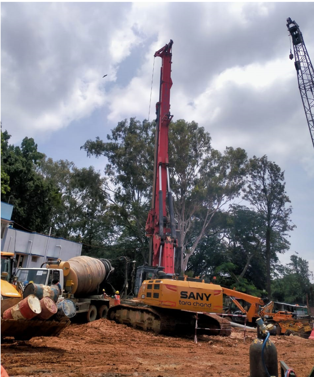
Our Piling Rig engaged at the BMRCL Bangalore Metro Project
