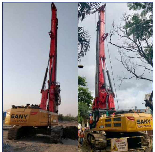
Piling Solutions at Infrastructure Projects
